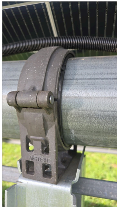
Figure 3 — the assembly, general view. The hinged Arctech bearing housing clamped over the black plastic bearing on the galvanised torque tube.
